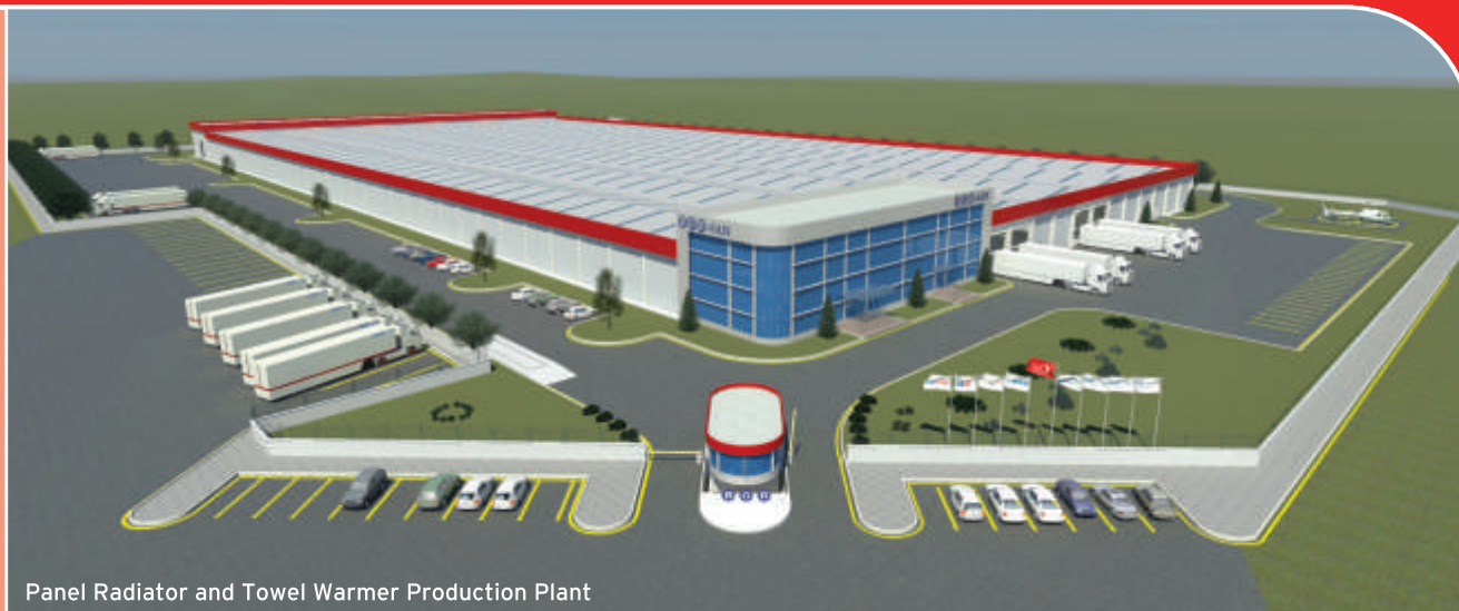
Panel Radiator and Towel Warmer Production Plant
